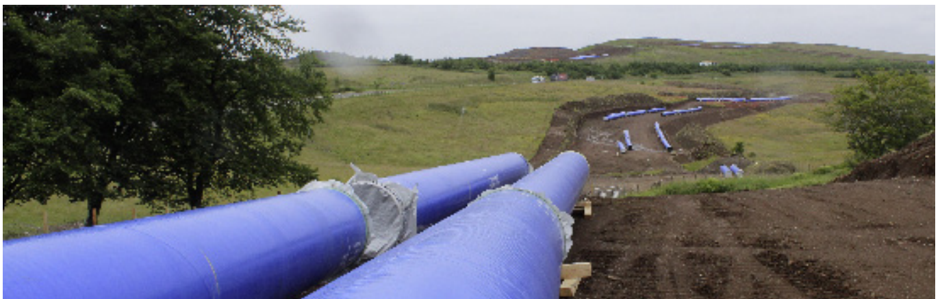
Amlaird pipeline gets ready for first connections
