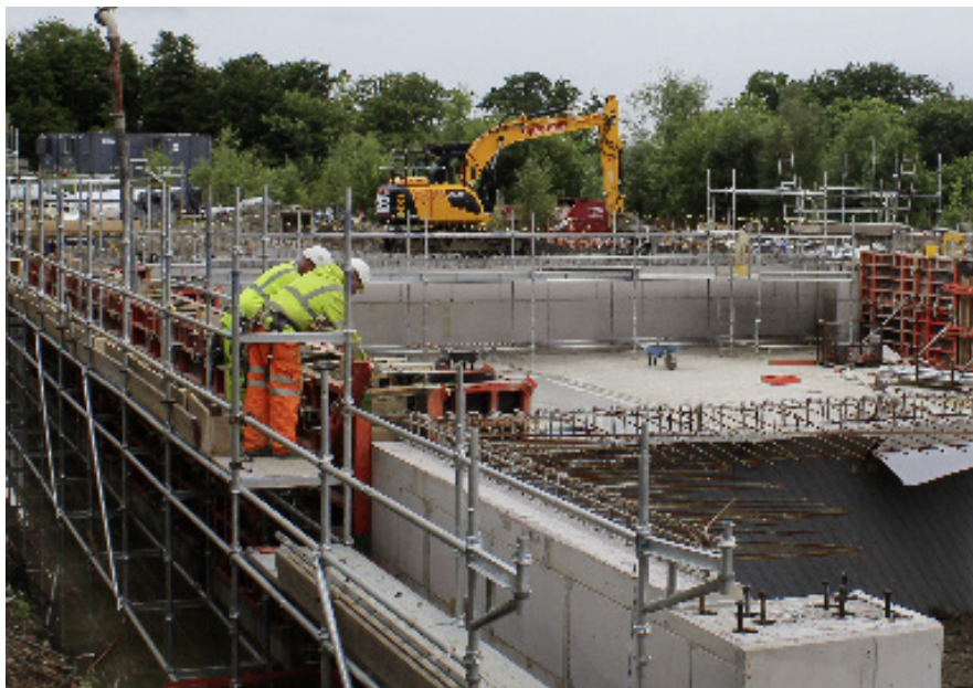
Building work starts on the new Corsehouse Pumping Station
