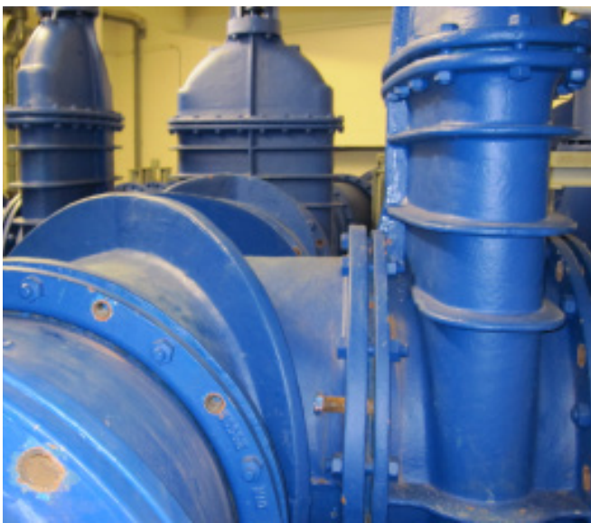
Valve room before replacement
