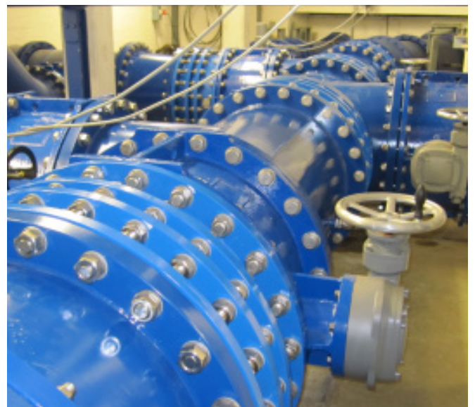
Valve room after replacement with AVK double eccentric butterfly valves in DN800
