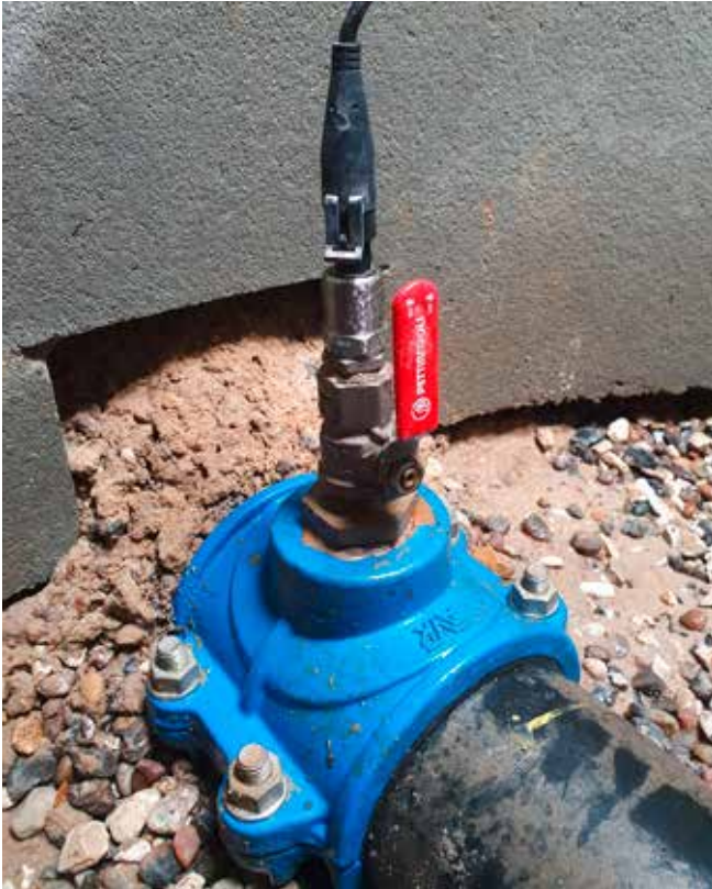
Due to the wireless nature of IoT, the pressure sensors can be installed at any critical point in the distribution network.
