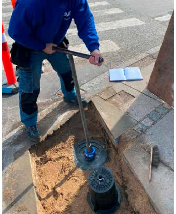
Underground gate valve with VIDI Positioner that detects when the valve is operated.
