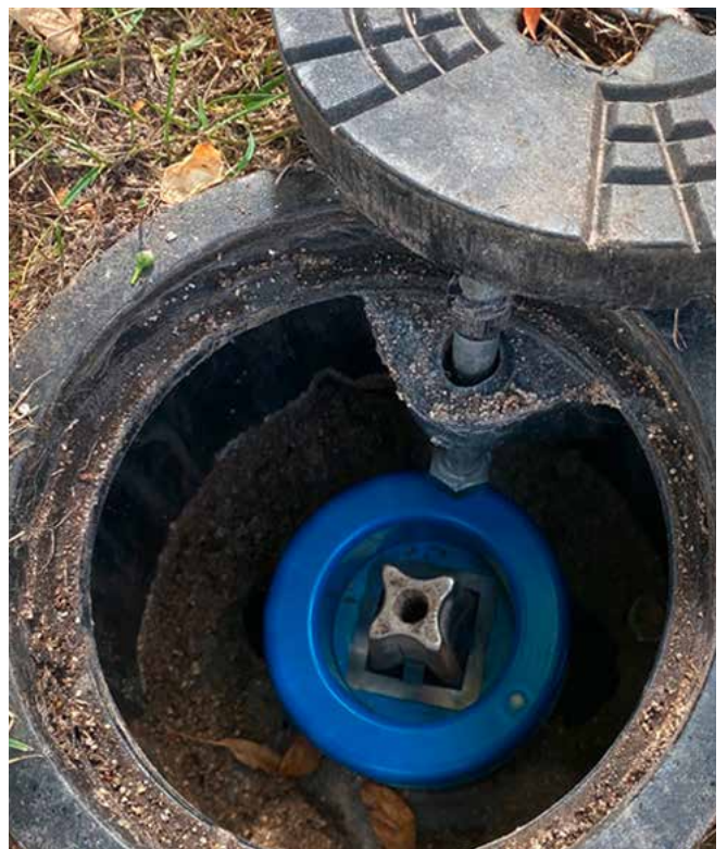
VIDI Positioner installed in a plastic surface box.
